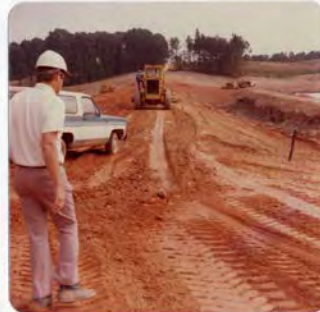
Placement of Material on dike.
